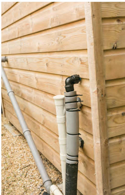
COMMERCIAL KITCHEN - Services
