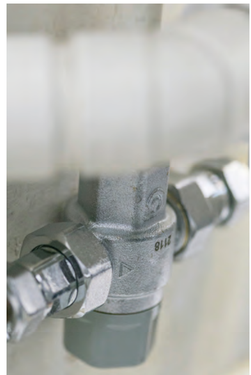
HEAT REGULATED VALVE - Pupil Safety
