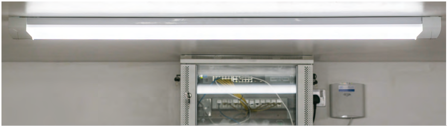
LED LIGHTING - Complete Upgrade to Energy Saving LED Fittings
