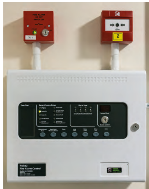
FIRE ALARM Install
