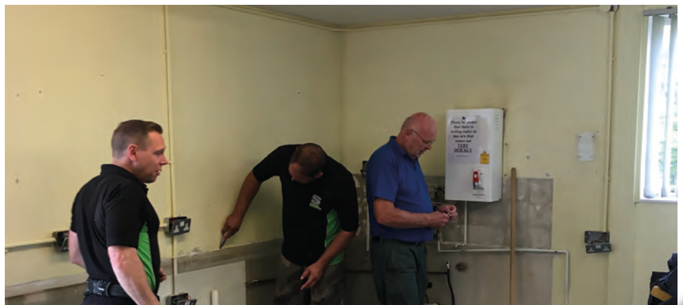
STAFF ROOM KITCHEN - Refurbishment
