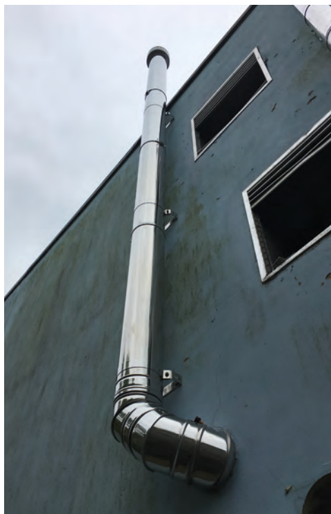
EXTERNAL BOILER FLUE - Installation
