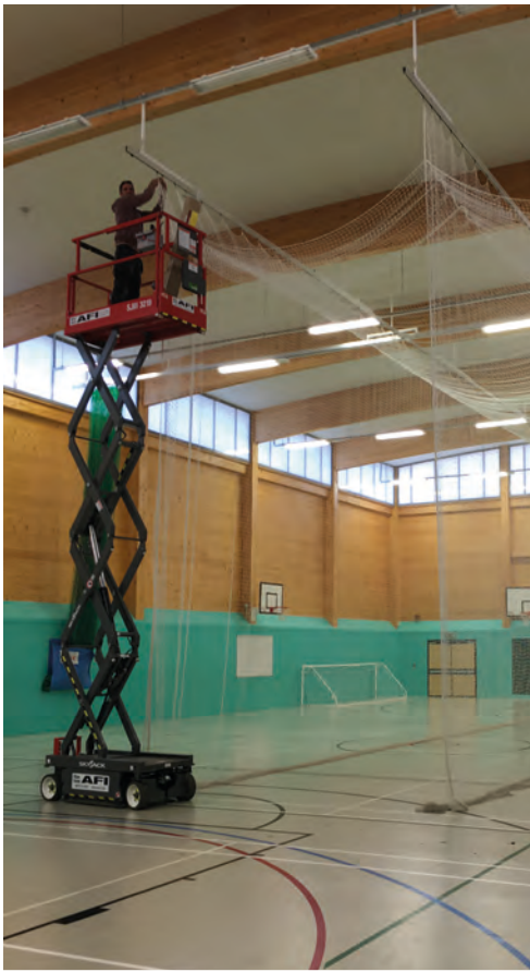
GYMNASIUM High Level Repairs
