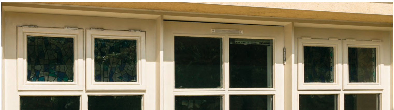
EXTERNAL DOORS - Full Repair & Decoration to all Exterior Windows & Doors
